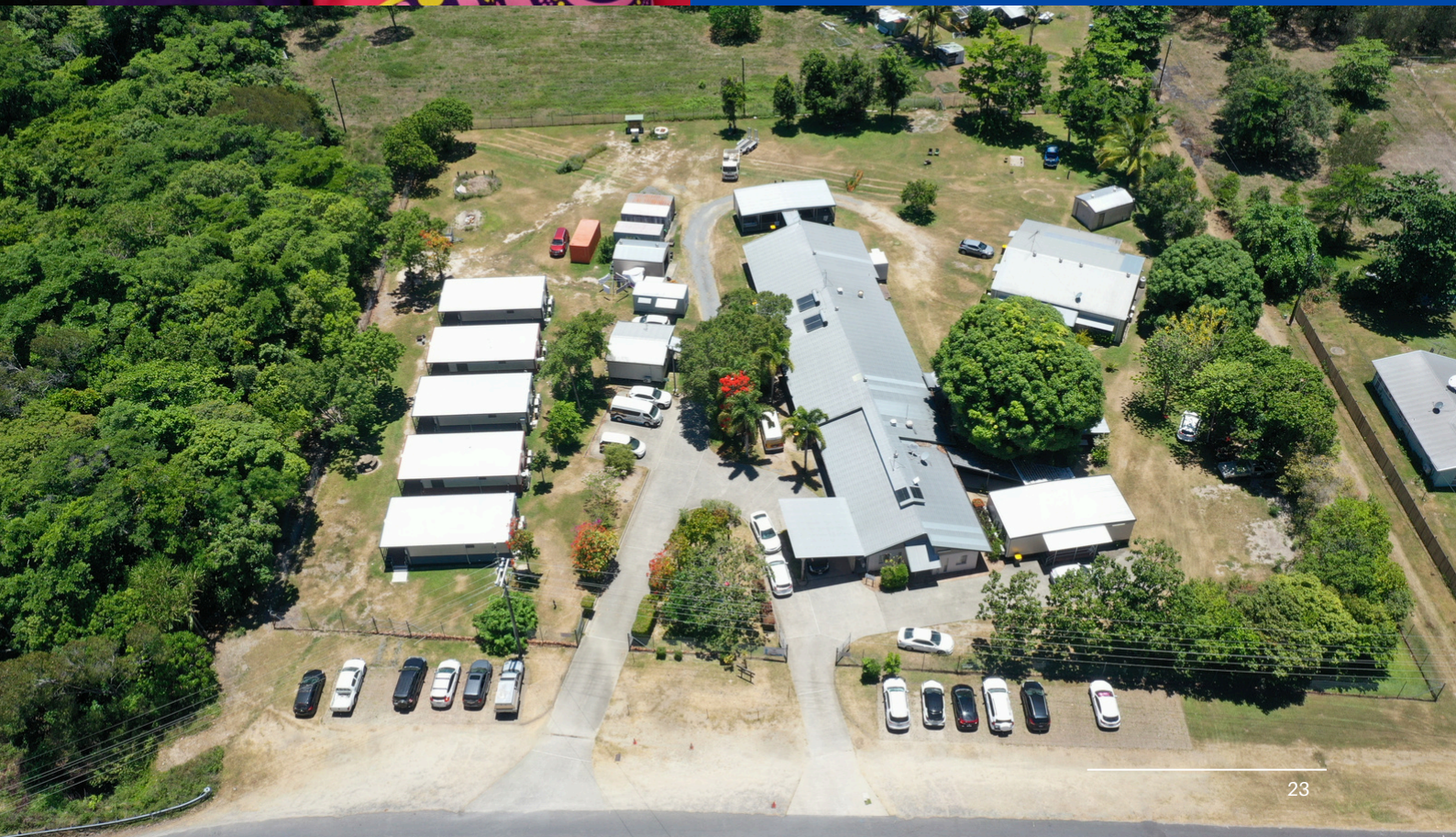
Below: Gindaja's Residential Recovery Centre in Yarrabah, which is currently undergoing an expansion to enhance its services and accommodate more clients.
